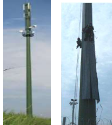
Mounting solution for CIGS flex module on cell phone towers
