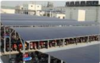
For carport roof
